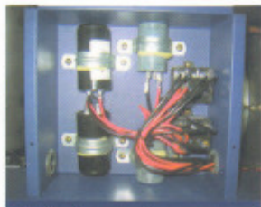
Start relays and capacitors minimize electrical load and reduce the energy
